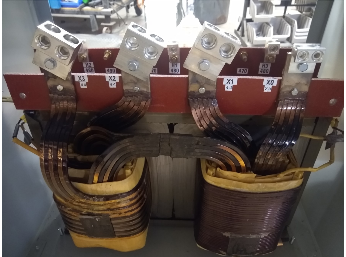
Transformer Primary (Back) and Secondary (Front) Connections
